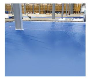
**ProctorGeo Gas Barrier 2000** is satisfactory for use as a gas-resistant barrier to restrict the ingress of radon, methane and carbon dioxide gases into building from landfill and naturally occurring sources.
