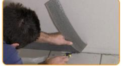
Lay down the final floor covering (ceramic or When the flooring application is completed, cut the exceeding part of the edging strips.
