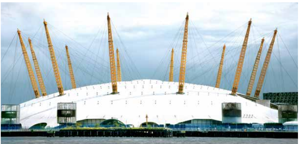
O2 Arena London (UK) – Arch. Richard Rogers
